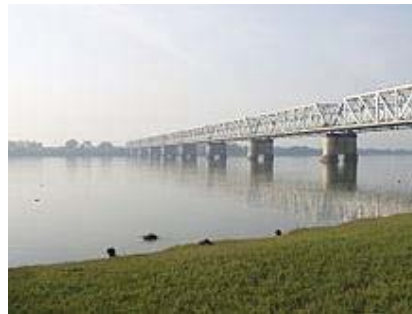
Fig. 1.4 Railway Bridge on river Narmada at Bharuch, Gujarat
